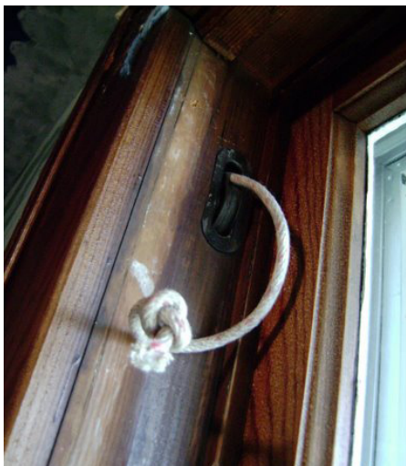
Pulley and New Sash Cord Photograph Series Courtesy of Slaves of the Vintage House
