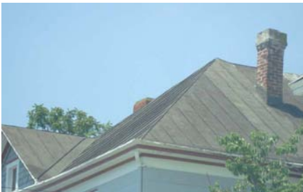
Metal Roof in Good Condition
