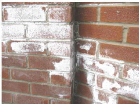
Efflorescence
